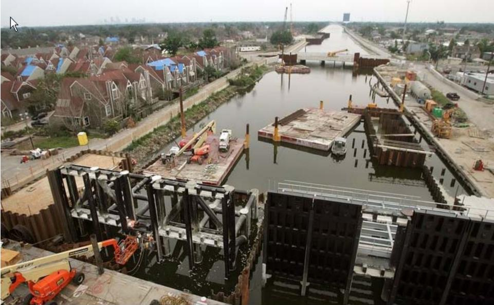
Work continues on the 17th Street Canal floodgates. The new Army Corps of Engineers plan considers building levees of between 30 and 60 feet in height to hold back water from severe storms.
