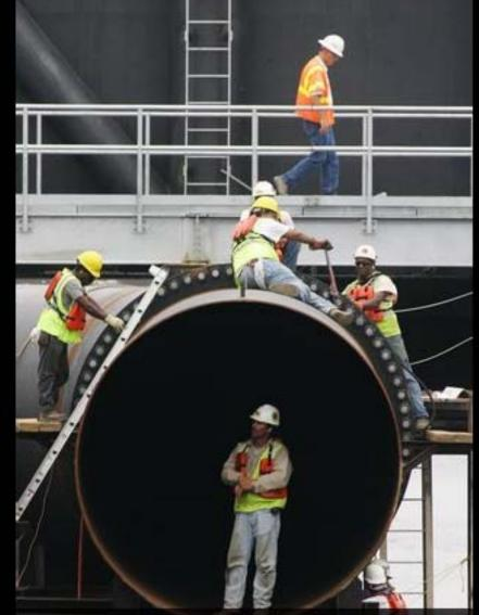
Workers install pipes to pump out water at the 17th Street Canal.
