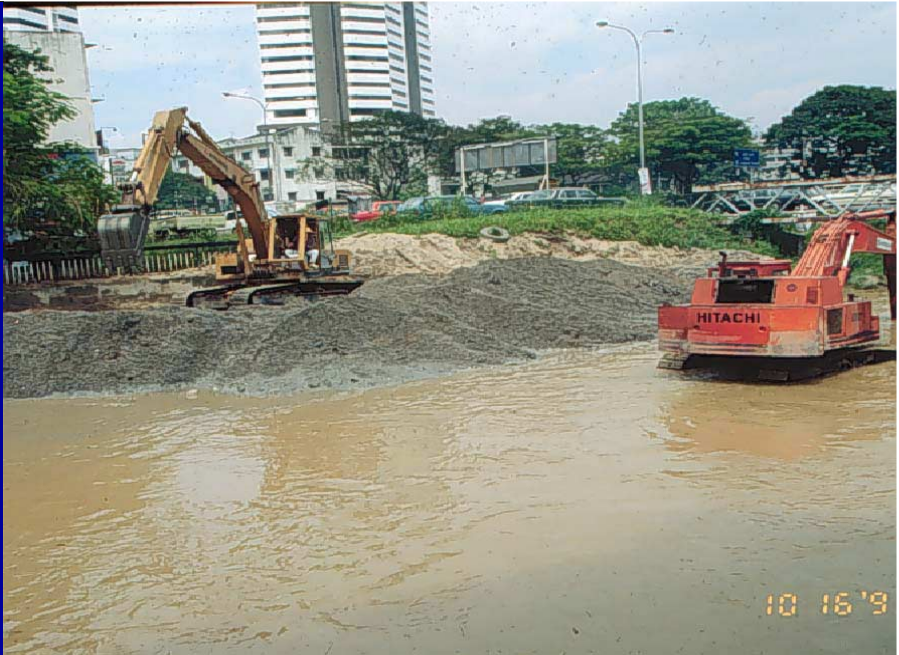
River Widening and Deepening
