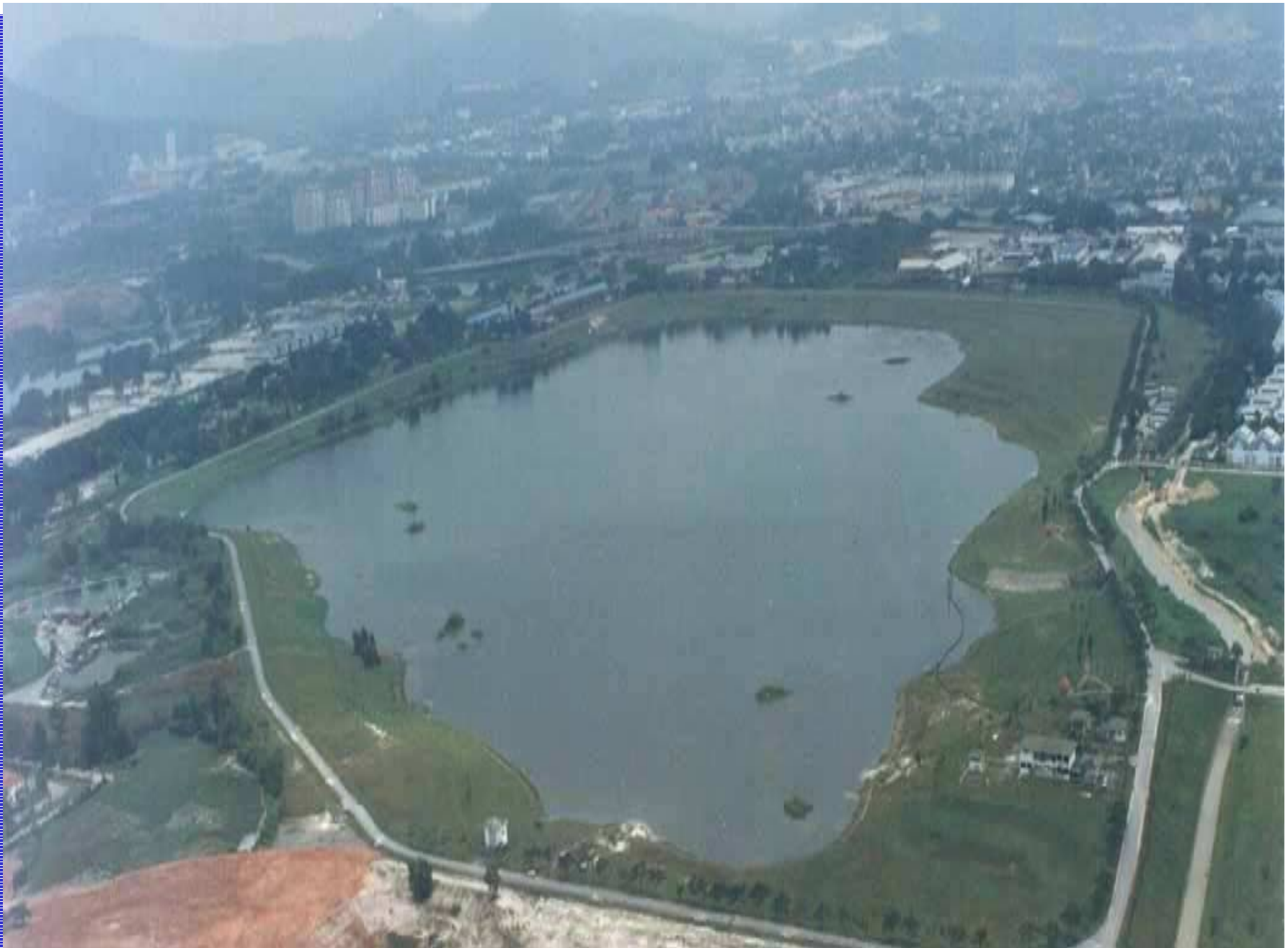
Batu River Flood Attenuation Pond
