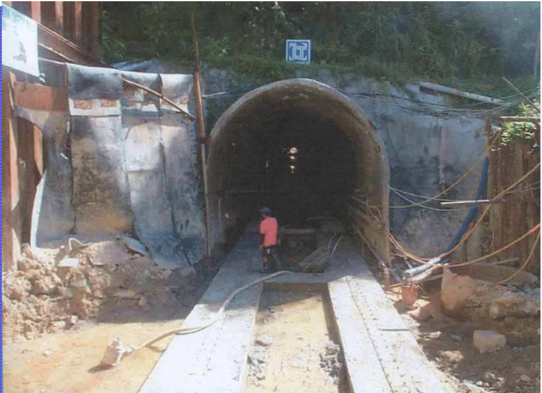
Sg. Air Terjun Flood Bypass Tunnel
