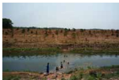
The breach point in the 1999 flood (In front of the river bank is an irrigation channel. The Baitaraini River runs beyond the bank.)
