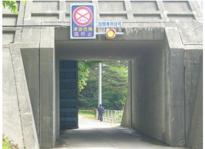
Photo3-2-2 Demonstration of the gate closing
