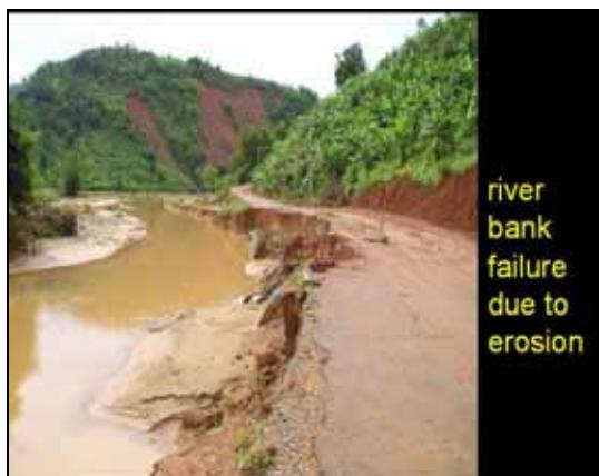
River bank failure due to erosion.
