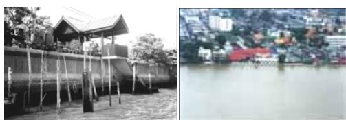
**Fig. 33 Flood Protection Walls (levees) along the Chao Phraya River**
