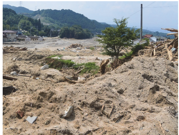
Landslide damage (photo by ICHARM)
