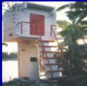
Water Level Station
