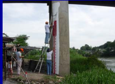
Installation of Water Level Gauge
