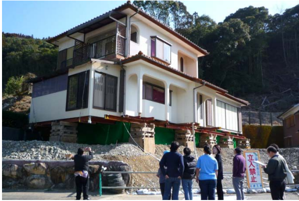
Explanation of the elevated house under construction
