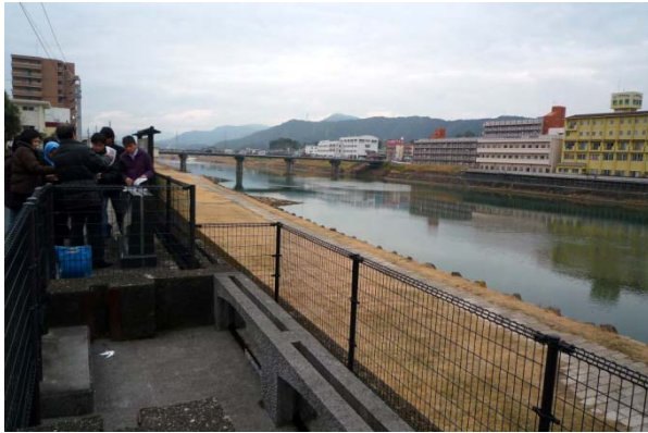
Tatami levee in Gokase River
