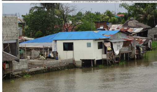
Detailed Hazard Map by ICHARM (top) and Flooding (bottom) in Calumpit, Pampanga River Basin, Philippines
